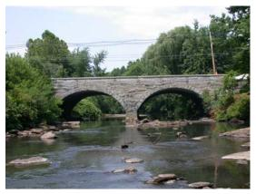
The Leominster Bridge is a two-span stone masonry arch bridge. The barrels and spandrel walls are constructed of gray granite laid in running bond. The spans are approximately 40 feet each and rise approximately 12.5 feet from spring line to crown. The bridge carries two-way traffic on Massachusetts Route 13 and has pedestrian walkways on both sides of the bridge.
