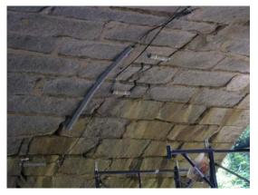
Numerous longitudinal cracks in the east barrel near the north spandrel wall were monitored using dynamic crackmeters.
